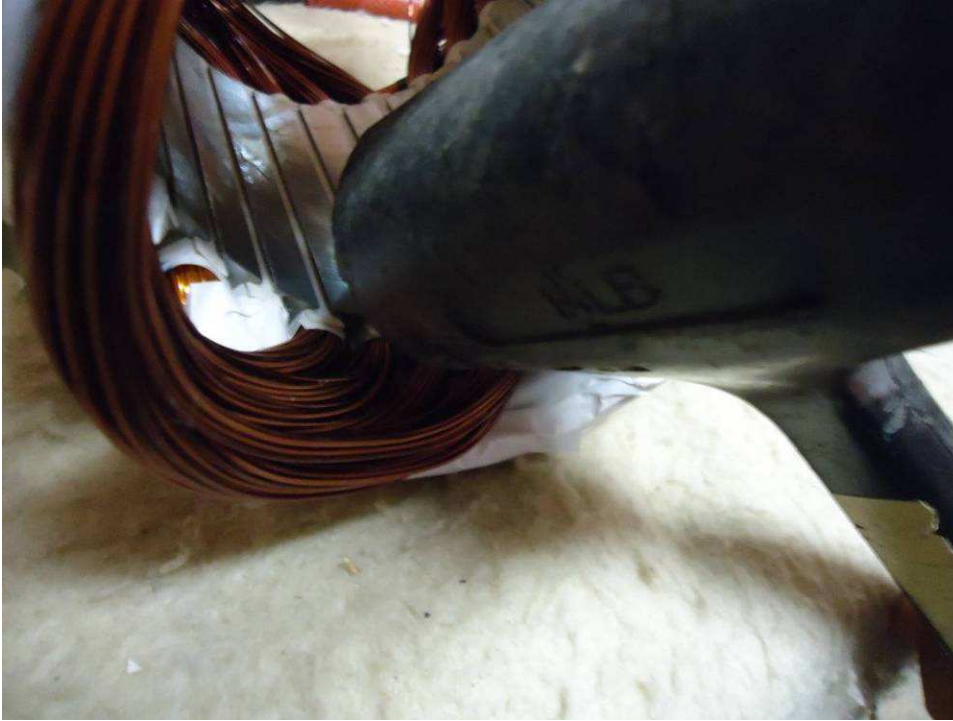
More taping the coils into shape.
